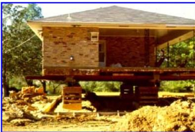
The aim of elevation is to raise the lowest inhabitable area above the BFE\*. Depending on the size of the house, the existing foundation structure, the magnitude of the expected hydraulic flood pressure and the raising level, this can basically be done by either extending the existing foundation or extending the exterior walls.
