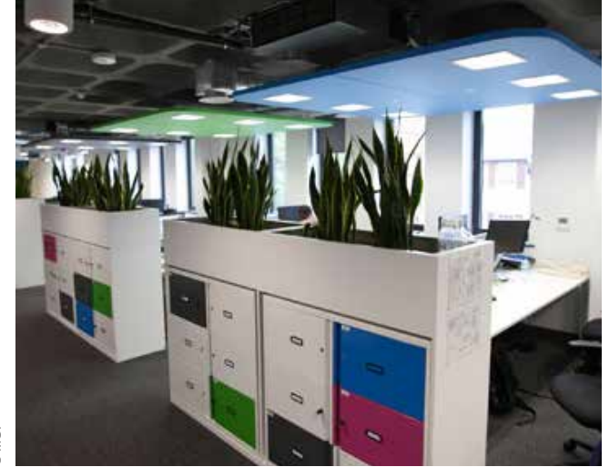
Philips 'pay per lux' high efficient lighting system at NUS building in London. The service model incentivises re-use of materials and design for long life
