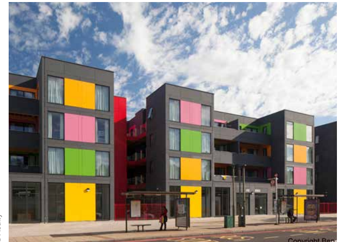
Modular volumetric construction for temporary housing at Ladywell, Lewisham. A rapid build solution that reduces waste generation. Also, units can be dismantled and re-used at another location.
