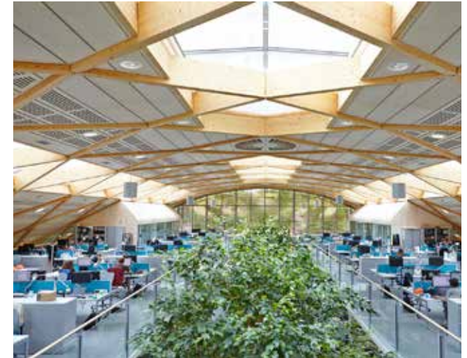
Low embodied carbon cross laminated timber structural members, WWF headquarters
