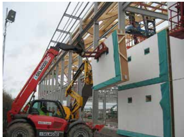
Hemclad wall panels at Marks & Spencer, Cheshire Oaks. A natural material embedded in modular panels which reduces operational energy and sequesters carbon
